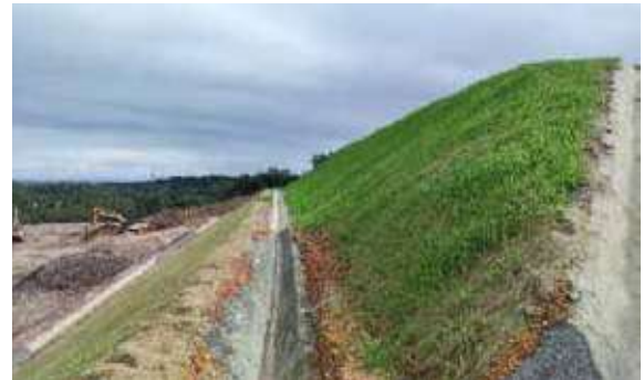
Silt fences and grass turfing are some of the environmental protection measures taken at MRSM Dungun
