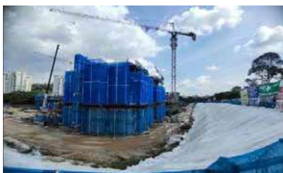
Implementation of geotextile for slopes protection at Sakura Residence
