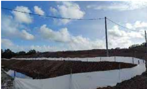
Silt fences and grass turfing are some of the environmental protection measures taken at MRSM Dungun
